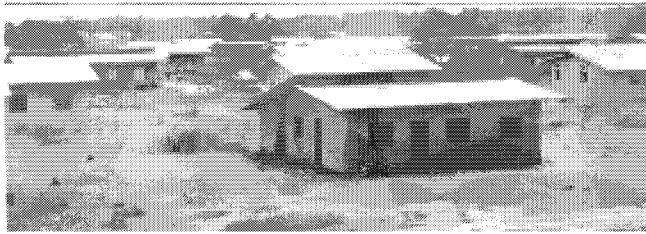
Losanganya housing project
